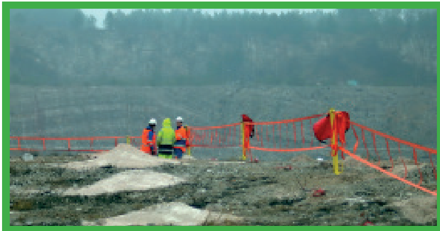
Barrier system at quarry face.
