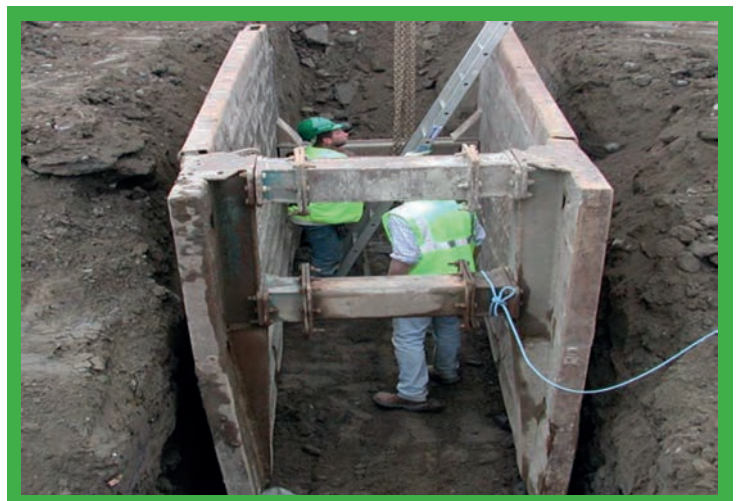
Trench Boxes in use.
