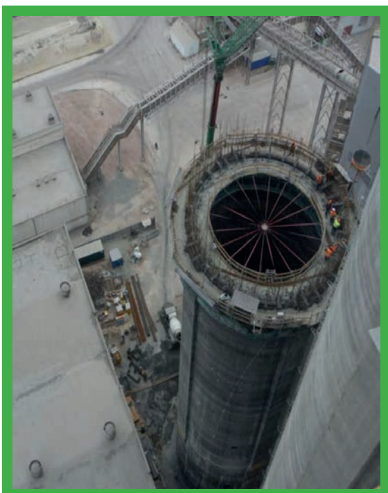
Raw Meal Silo Project.
