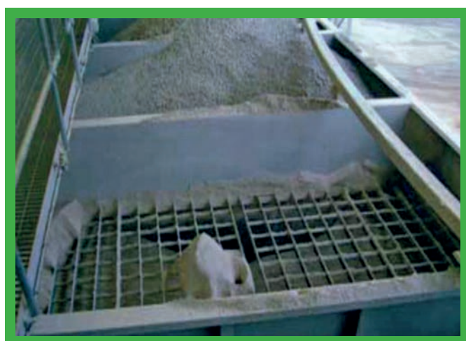
Man grids in place.
