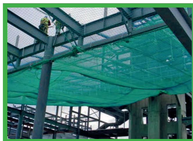
Safety Nets in use.
