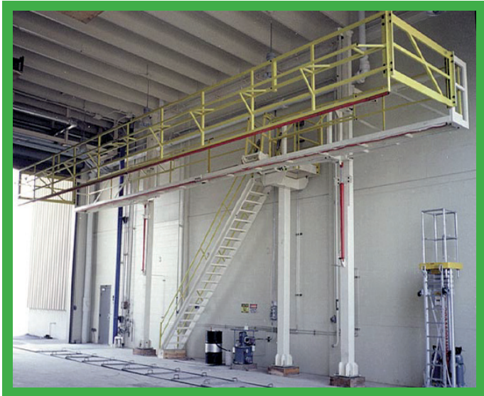
System at Finnsementi to protect the tanker driver during loading. This system has to be adjusted in terms of length and height to cover all vehicle sizes.
