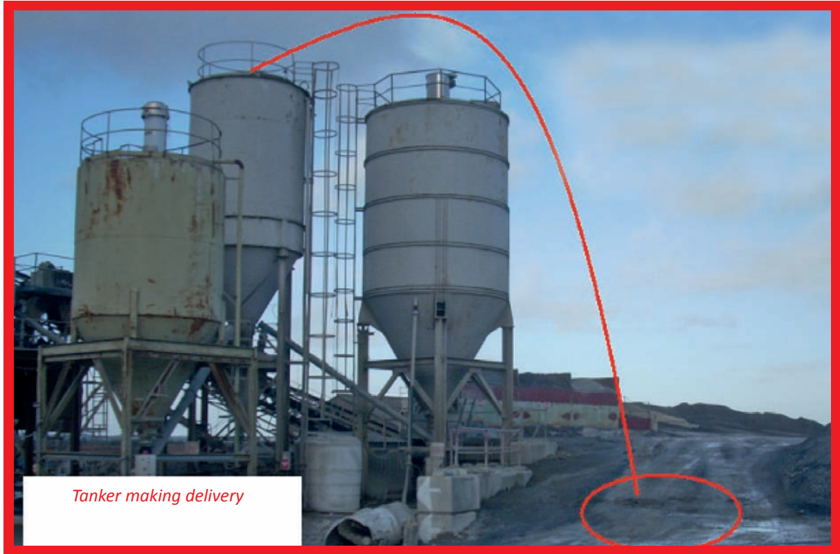
Incident - Near Miss 2019: Filter blown onto nearby area
