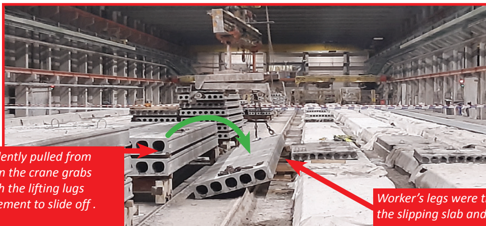
When the slab was lowered into position - the operator released the grabs / clamp and lifted the clamps higher upward to move them away from the next task.
