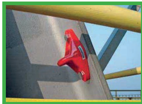
Additional securing hooks for harness use - installed where required.
