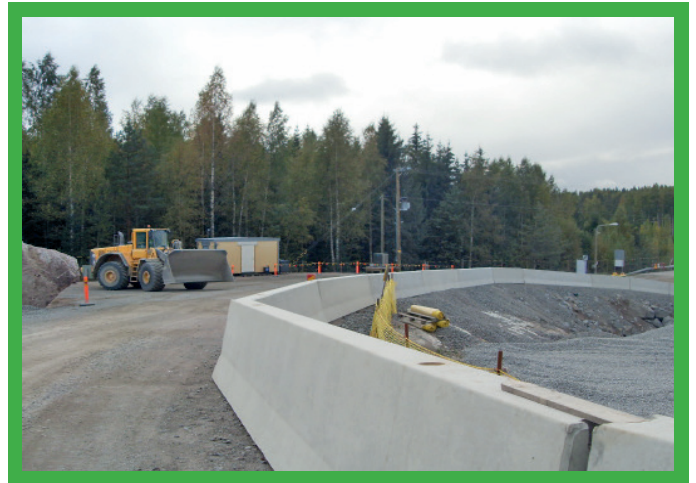
Edge Protection using precast structures.
