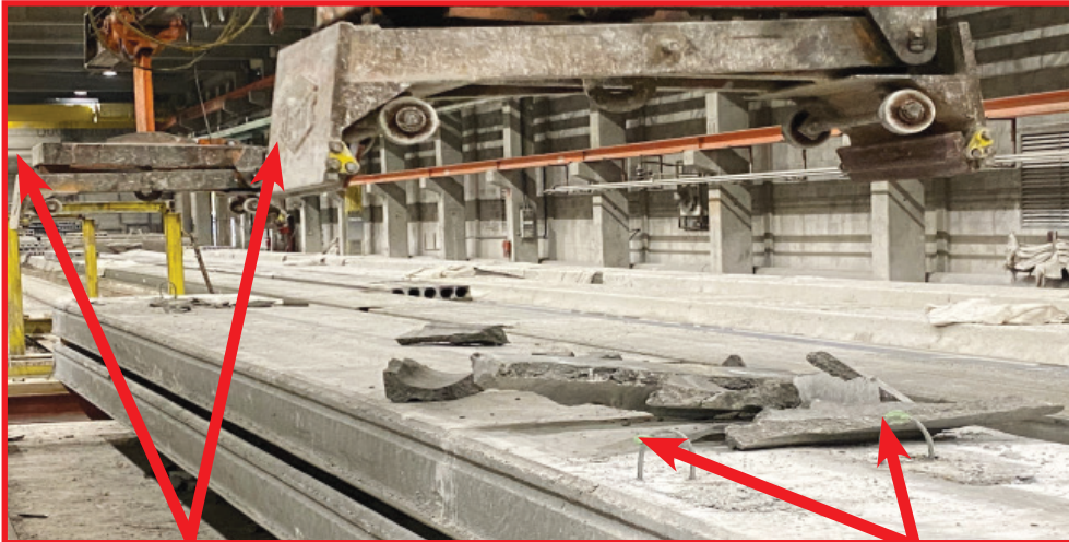
Hollowcore slab is lowered into position using the clamps / grabs from an overhead crane.
