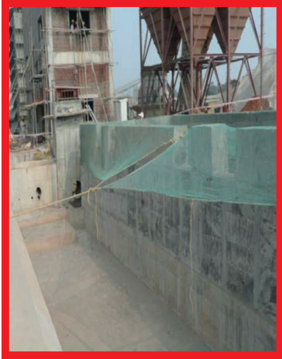
Fatal Accident 2011: Contractor fell while crossing a wall during the construction of an extension.
