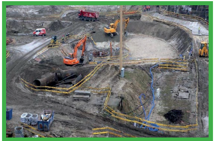
Transport systems at a construction site.
