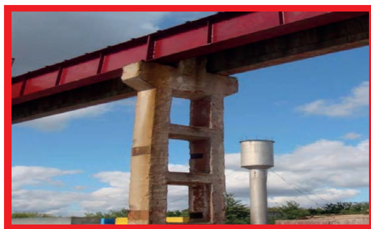
Group Fatal Accident - Case Study 2008: Contractor fell from upper level while descending. Risk assessment identified the need for a MEWP (Mobile Elevating Work Platform), but none was used.
