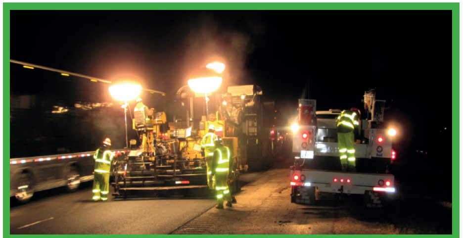
Road-surfacing at night close to live traffic.
