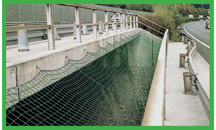
Safety Netting in place.
