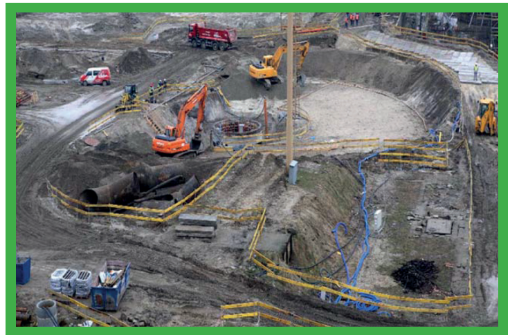
Transport systems at a construction site.
