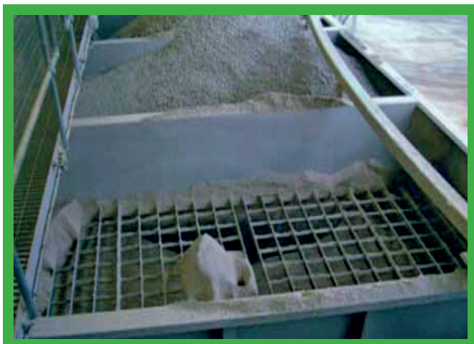
Man grids in place.
