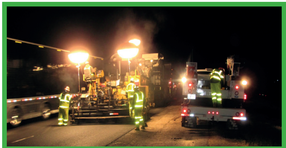
Road-surfacing at night close to live traffic.
