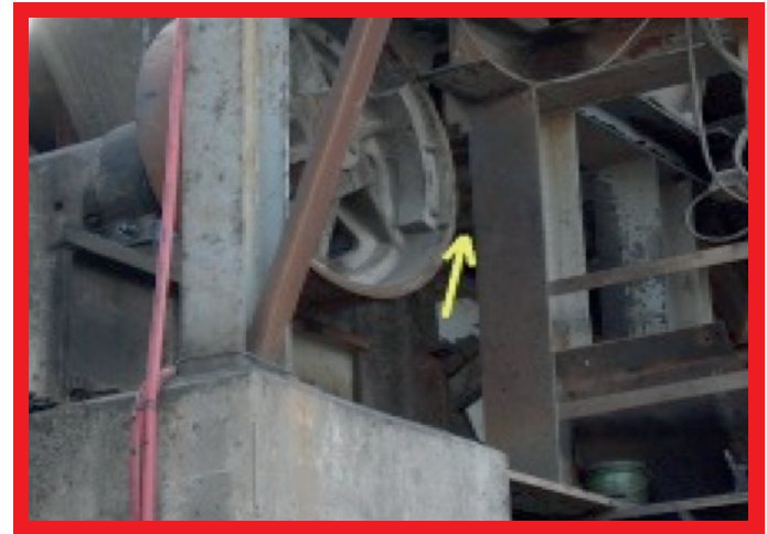
Group Fatal Accident - Case Study 2006: During a lifting operation, a supervisor was trapped between the load being lifted and a steel beam.
