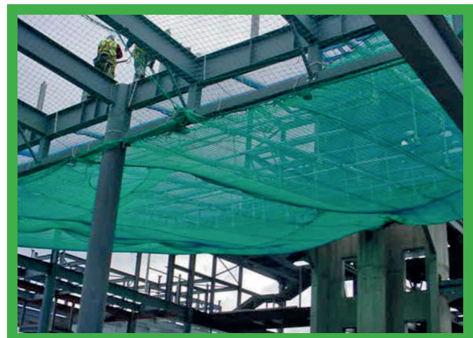
Safety Nets in use.
